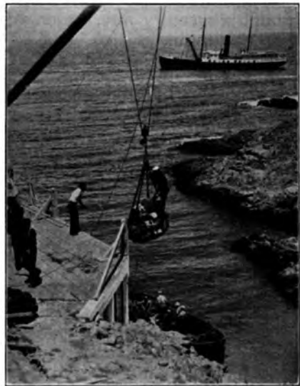
Landing Supplies Under Difficulties
